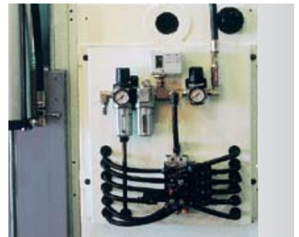
Pneumatic parts in one plate easy to inspect and maintain.
